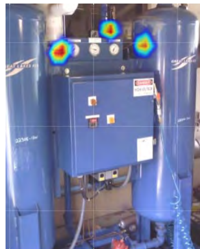
Figure 1. With portable acoustic imagers, technicians can quickly locate compressed air leaks simply by pointing the device at an asset or system or scanning a large area – from a safe distance, with the line still running, and no matter how noisy the plant.
