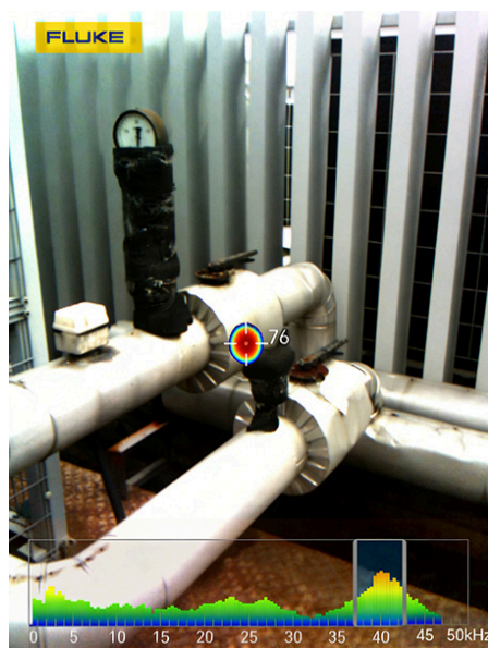
Leak detection on a pipeline
