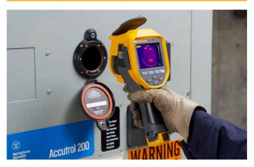
Thermal imaging or infrared imaging has become commonplace in most daily plant operations. As the number of infrared scans increases, so too does the exposure to and risk of arc flash. Enclosures must be opened to scan with infrared (IR) and doing so greatly increases the likelihood of an arc flash explosion. IR windows can mitigate this risk by allowing infrared scans to be performed without opening enclosures, virtually eliminating the risk of an arc flash.
