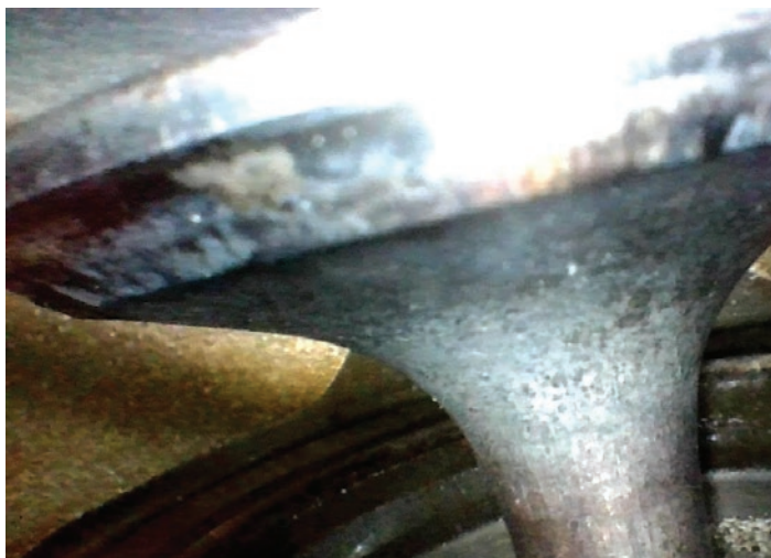
Photo above: Valve inspection
